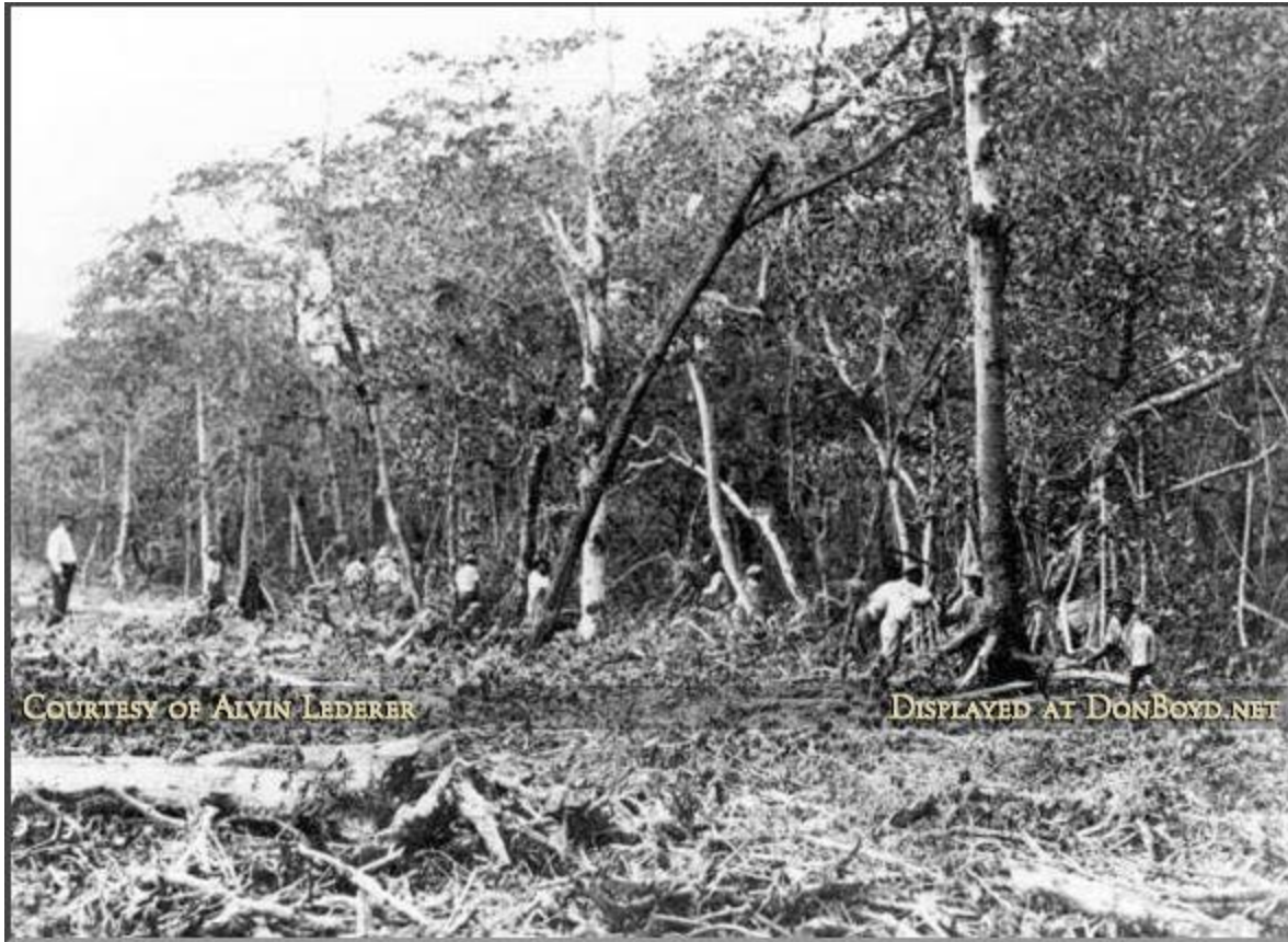
1910s – Workers clearing every mangrove from Miami Beach. Photo by Don Boyd
